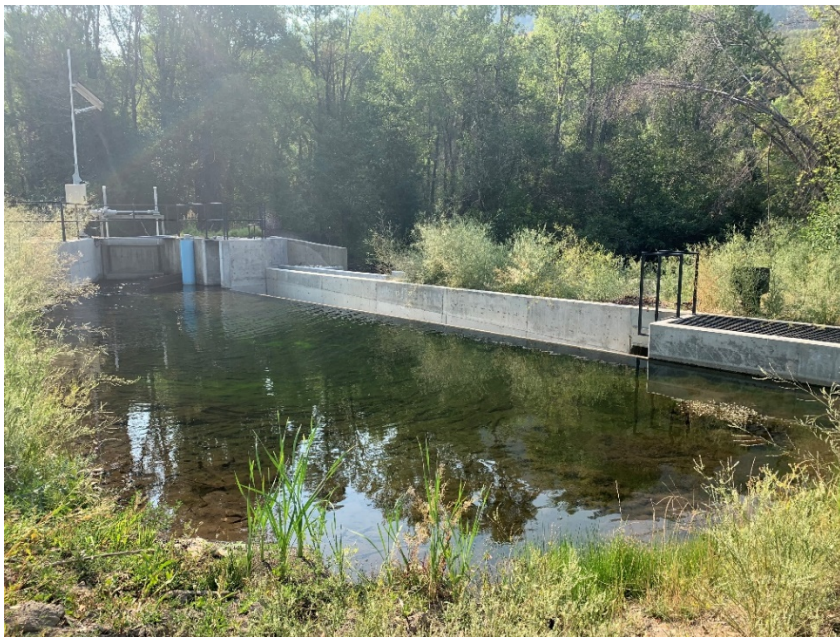
Figure 9 – Needle Rock Ditch Company new pipeline screening structure, stilling basin and fish passage. Flow is from left to right. The SCADA installation with mast and solar panel can be seen to the left of the new headgate entrance, Crawford.
