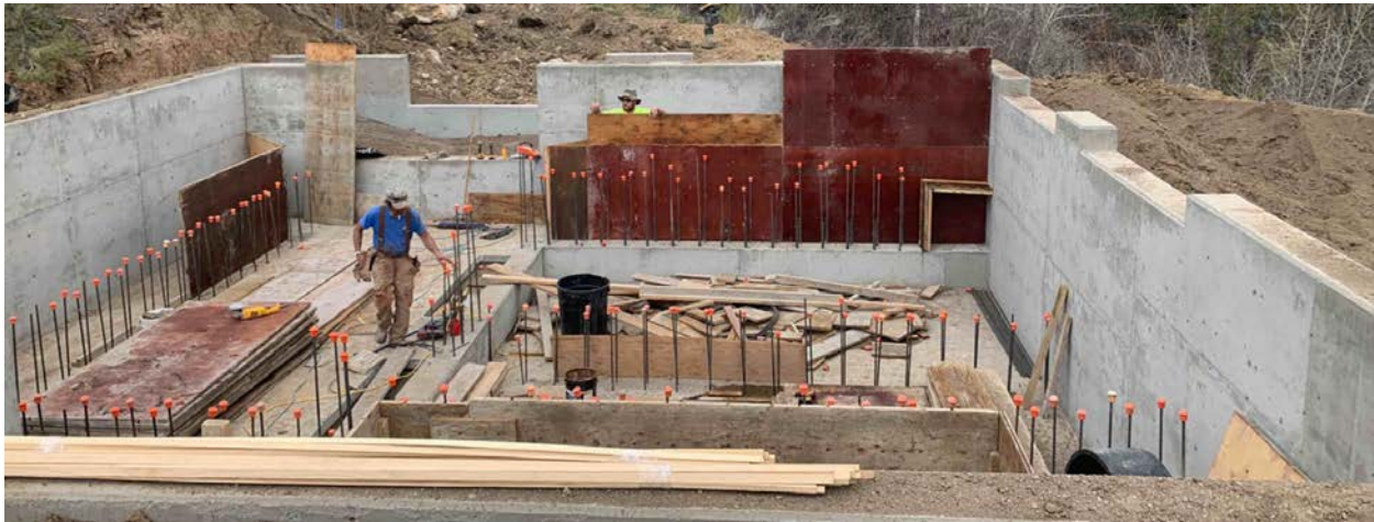
Figure 12 – Grandview Canal inlet and screening structure during construction, Crawford
