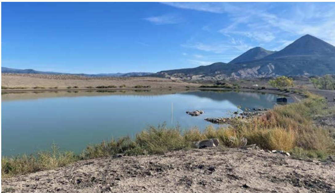
Figure 6 – The completed 4C regulation reservoir after construction, near Crawford, Colorado.
