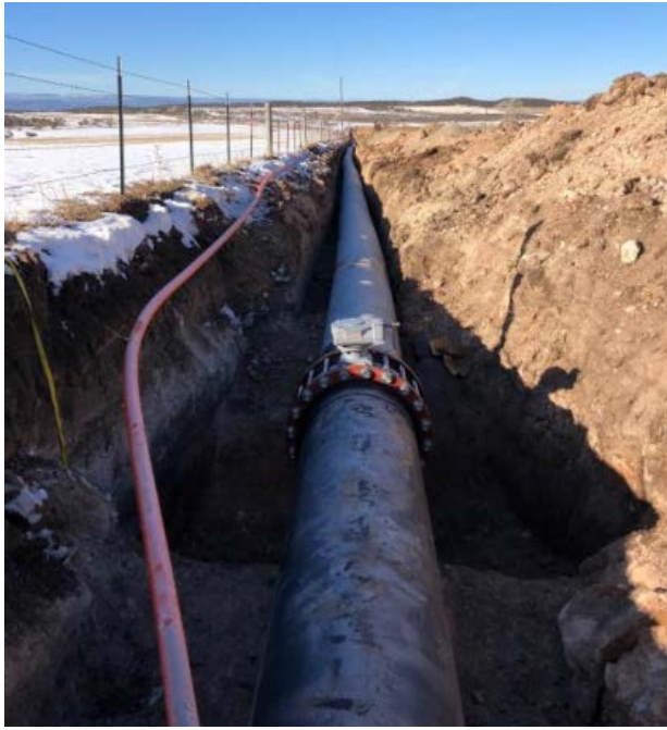
Figure 14 – Bostwick Park West Lateral Improvement Project showing piping and valve installation
