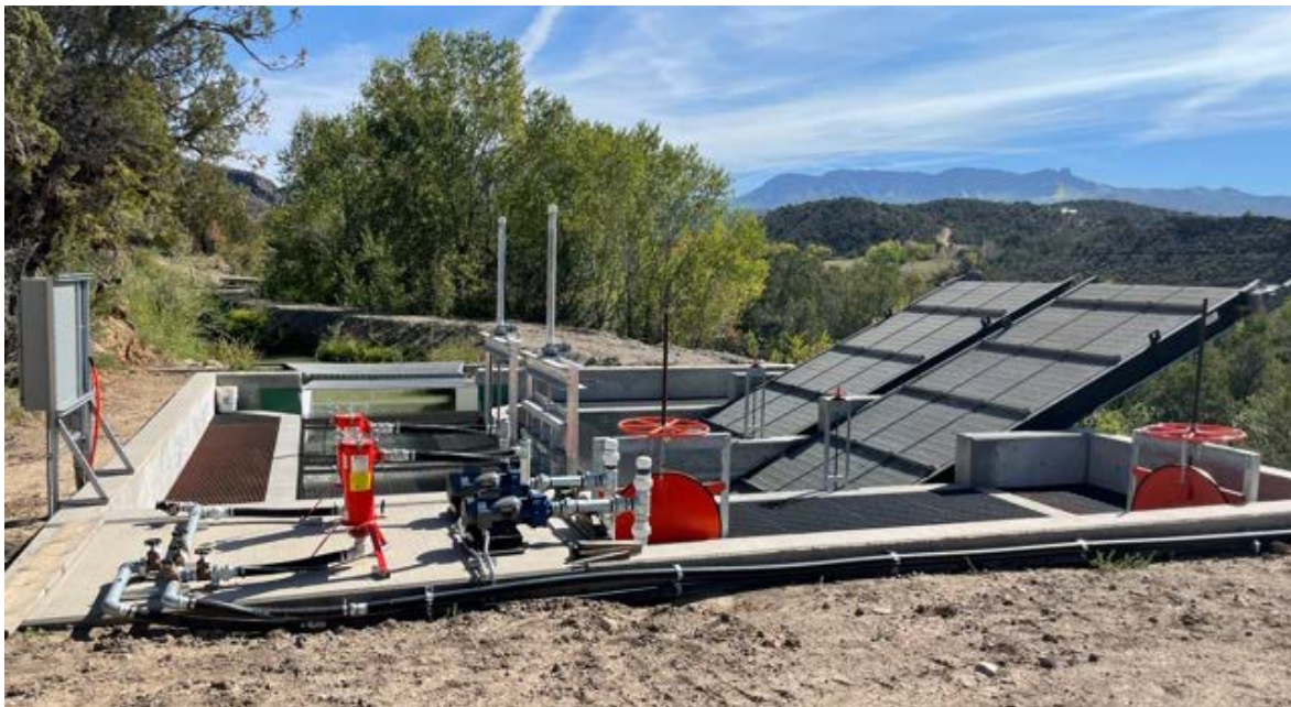
Figure 13 – Grandview completed canal inlet and screening structure, Crawford, Colorado
